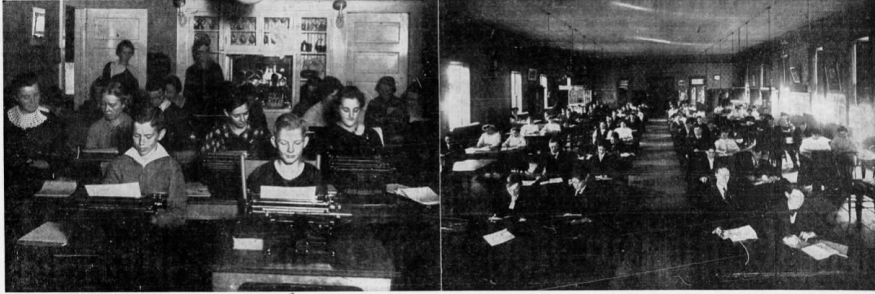
During the earthquake, which damaged the building housing the Helena Business college, Mrs. D. P. Patenaude, manager, moved the entire plant to her residence where school was resumed promptly. The earthquake caused the building to be destroyed in 1917, and the school was moved to the Higgins building on Flavel, where it has been located since.
